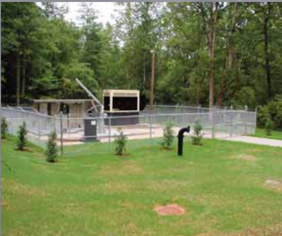
The newly constructed pump house at The Settings of Lake Rhodhiss.
